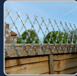
Razor Mesh on Fence Topping
